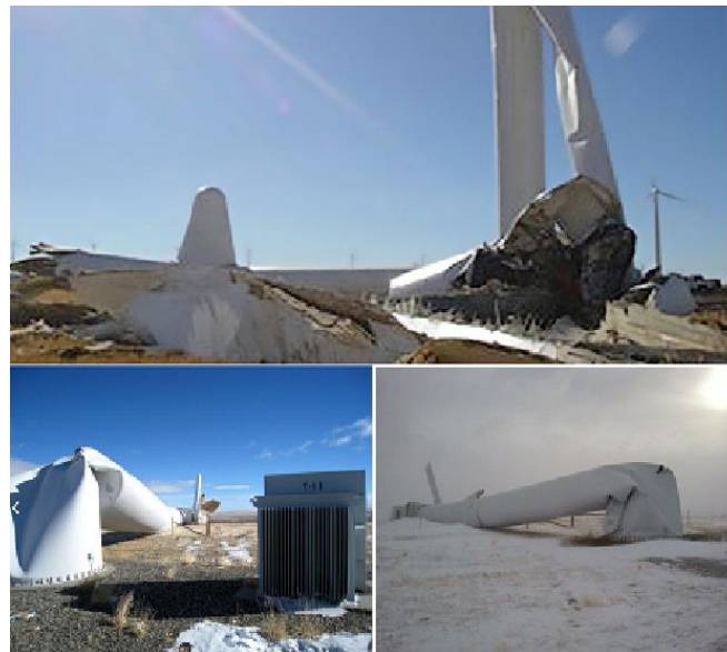
Fig. 1 Failure of steel wind tower (Khatri 2013; http://galleryhip.com ; Ruralgrubby's Wind Watch)
